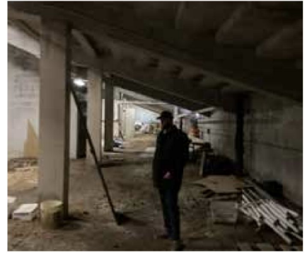
Space Under Grandstand
